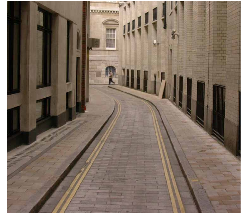
Retained raised kerb to carriageway
