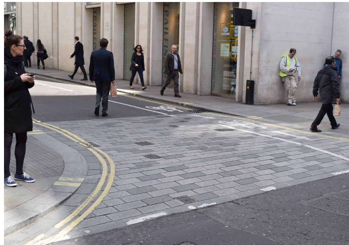
Granite setted courtesy crossing
